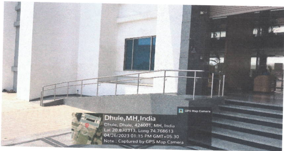
Geo-tagged photographs of the Ramp facilities for the year 2022-23
