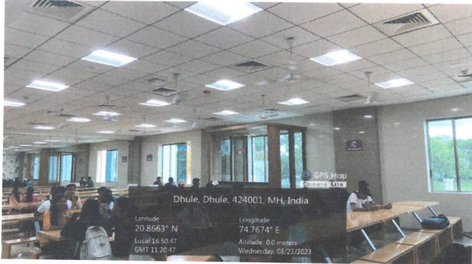
Photo. LED lighting in canteen – 23/08/2023
