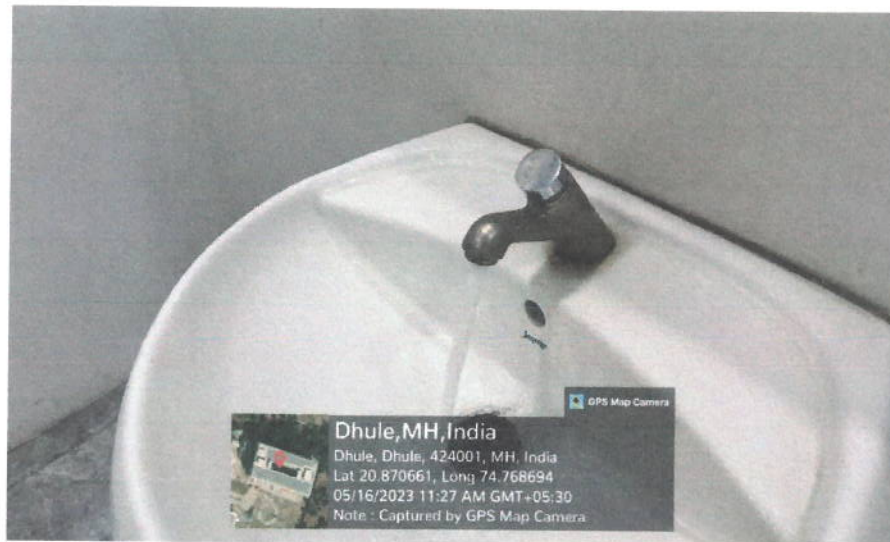
Photo. Automatic tap shutoff for water conservation – 16-05-2023
